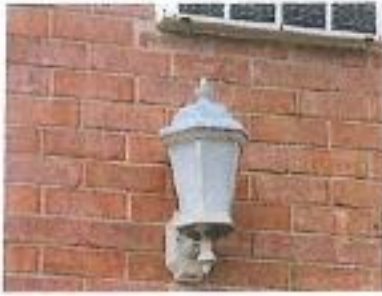
Exterior Lighting 02.jpg
