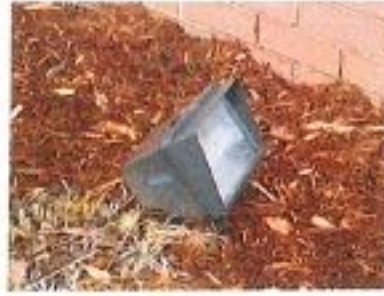
Exterior Lighting 03.jpg
