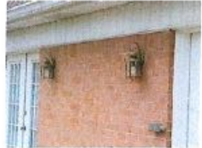
Exterior Lighting 01.jpg
