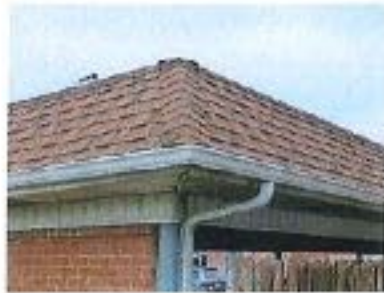
Gutters & Downspouts 01.jpg
