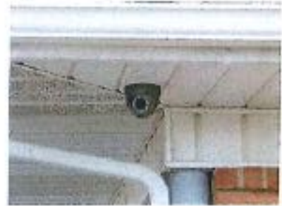
Gutters & Downspouts 02.jpg
